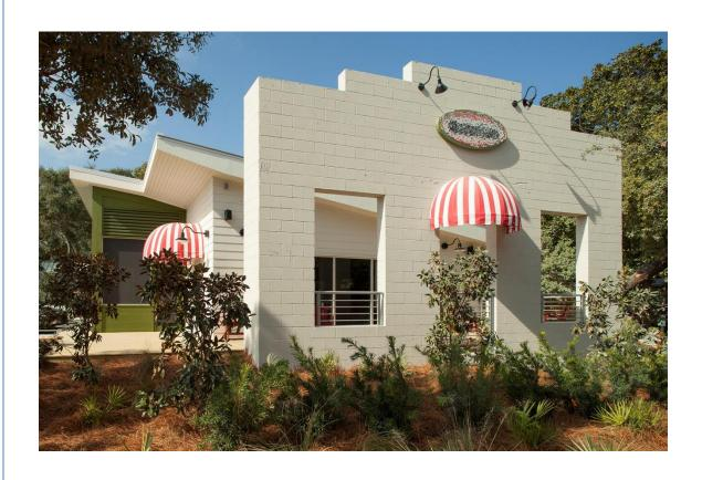
A mix of materials is used: painted block, pressure treated wood, and hardie siding.
